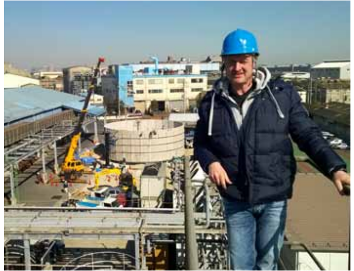
EnviTec Project Manager Andreas Bosse in front of the plant under construction.
