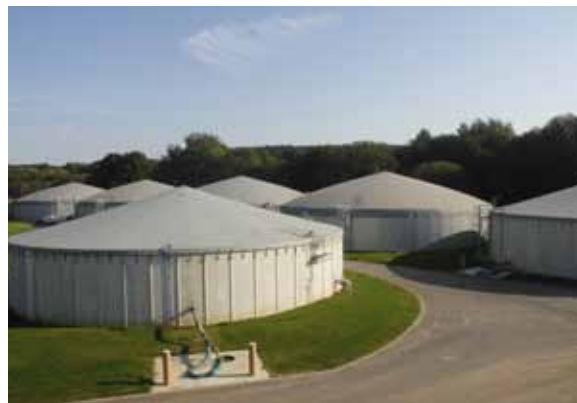
EnviTec own plant operation in Libramont: excess energy is fed into the national electricity network
