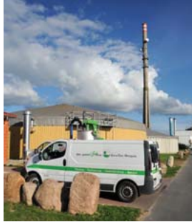
The plant feeds just under 1.6 MWh per hour into Cofely's heat grid.
