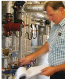
Farmer Johannes Seneca supplies the old people's home with heat all year round.
