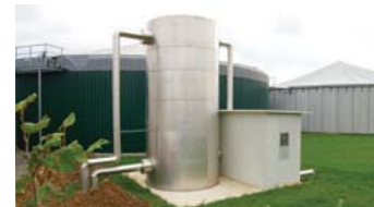
The heat tank contains sufficient hot water for the district heat network.
